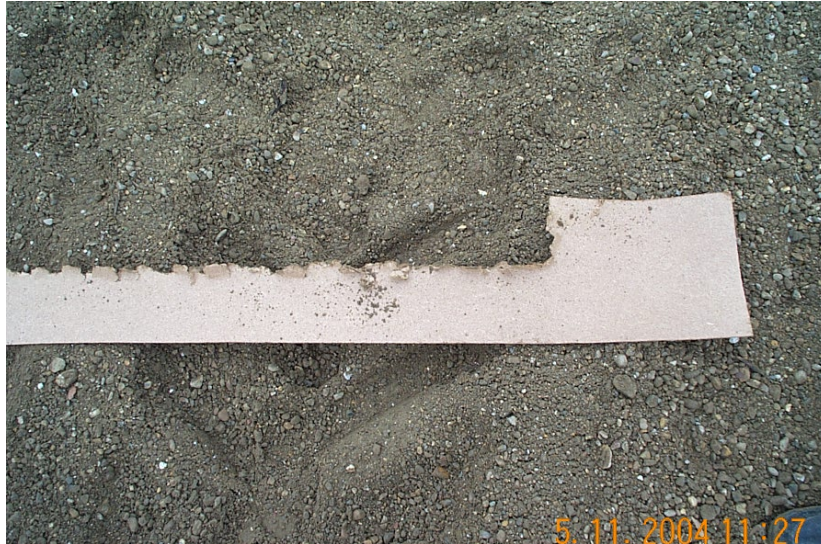
Figure 22 – Damaged fiberboard on the gravel lane
