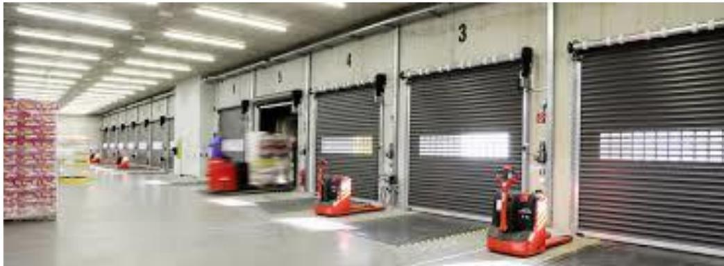
VIP2 dock levellers offer you the possibility to bridge the difference in height and distance between the warehouse floor and vehicle in the most efficient way.
